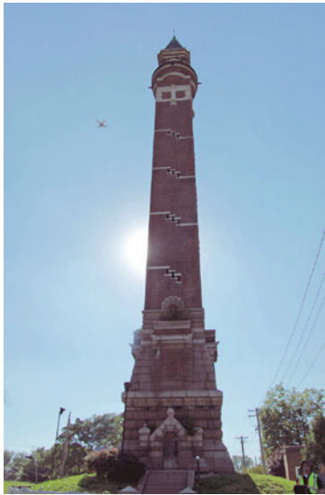
The Red Water Tower being surveyed by drone, upper left.
